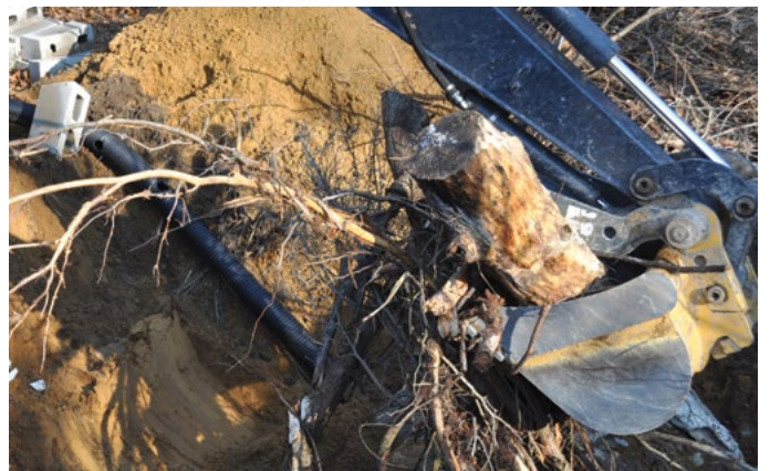
Figure 13. Some woody material (e.g., roots and stumps) should be included in the hibernaculum construction but their quantities should be limited to guard against excessive settling over time. © G. Beck
