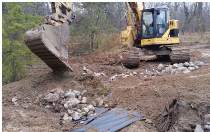
Figure 14. Landscape fabric placed across parts of the top of the constructed hibernaculum and covered with rocks, logs and topsoil to form a mound provides additional insulation. © G. Beck
