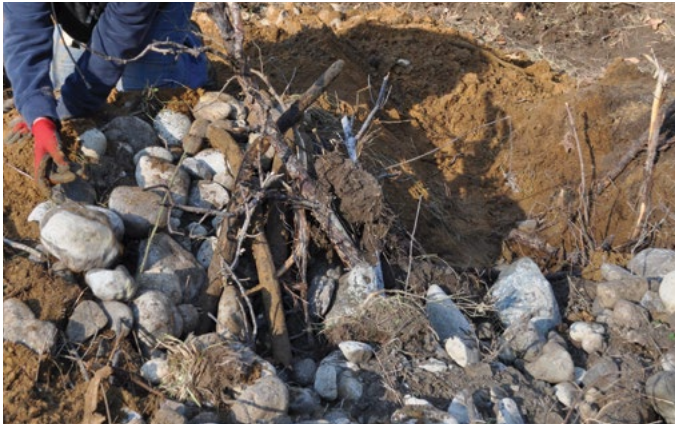
Figure 16. Brush and field stone cover the entrances to the pipes at the surface, providing cover and insulation. © G. Beck
