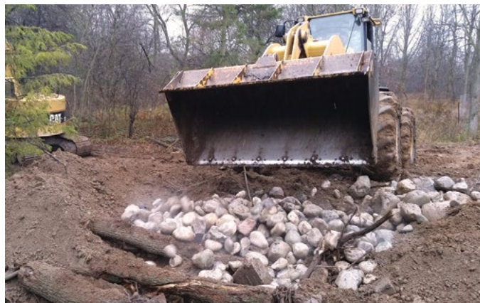
Figure 15. Field stone, brush and stumps near the surface provide hiding and basking sites for snakes and potential access points into the hibernaculum through inter-connected underground passageways. © G. Beck
