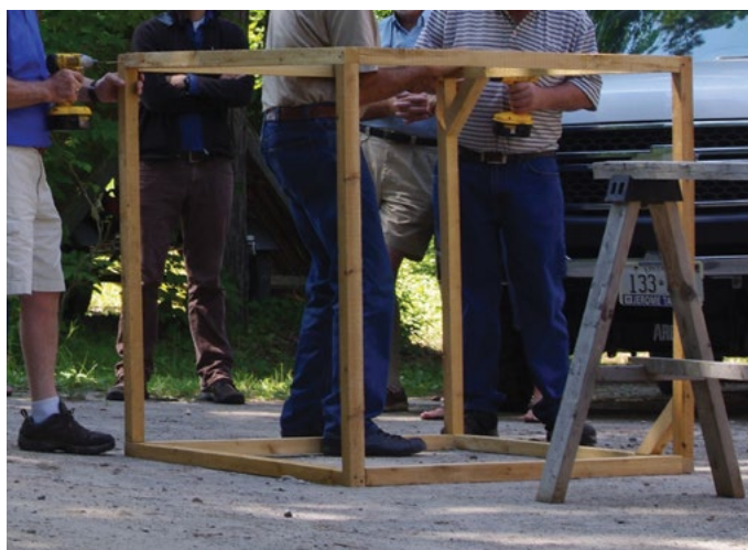
Figure 19. Assembling a nest box for Gray Ratsnakes. Corner braces are visible in two of the corners. © B. Barkley
