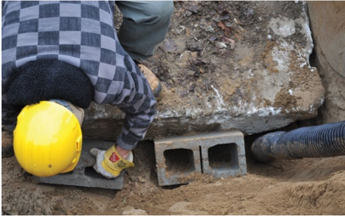
Figure 9. Use construction blocks to create chambers near the bottom of the hibernaculum and to keep concrete slabs from lying flat against the bottom or one another. © G. Beck
