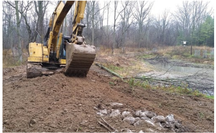
Figure 17. Final grading away from the openings ensures that surface drainage will not lead to potential flooding of the hibernaculum. © G. Becks
