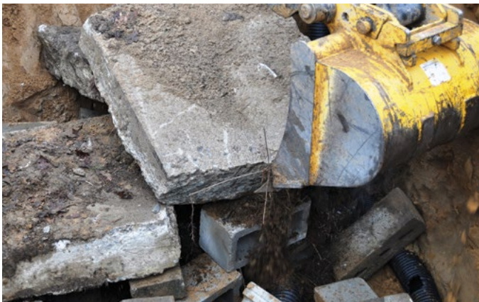
Figures 10 and 11. Position materials carefully to create inter-connected passageways and deep chambers. © G. Beck
